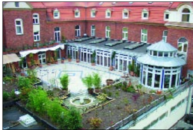
The open-air dance venue shortly after completion: 200m 2 dance-floor and 300 m 2 of garden.
