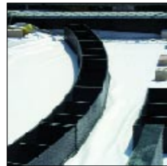
Curved APP Planting-Troughs were used as a boundary around the pavilion
